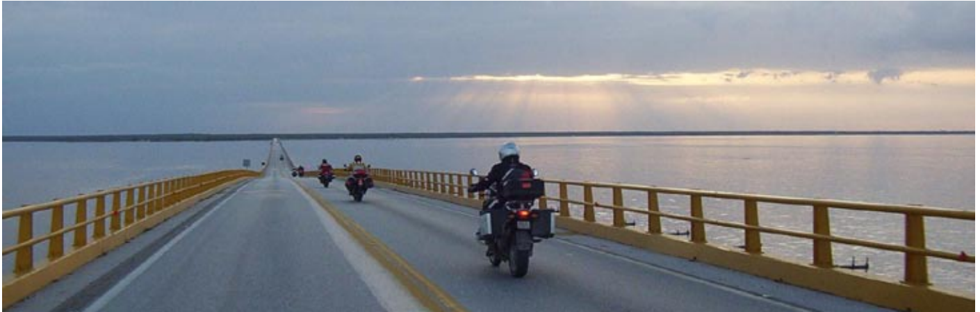
Crossing the bridges of the Gulf of Mexico
