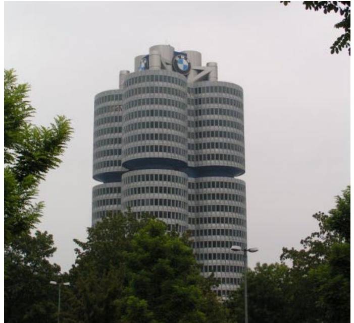
"4 cylinders" – BMW Headquarters in Munich
